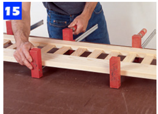
15 Use three or four clamps to squeeze the front rail assembly, pressing the slats to the bottom of the mortises.
